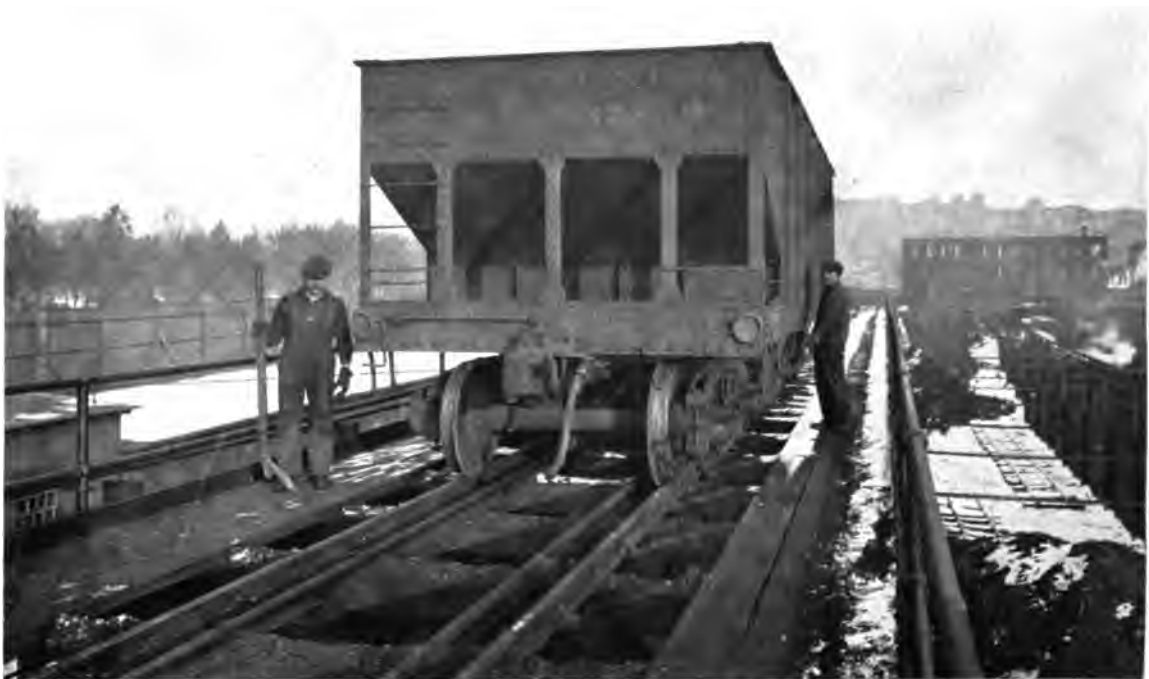
Fig. 1. Footwalks on Coal Trestle.*
